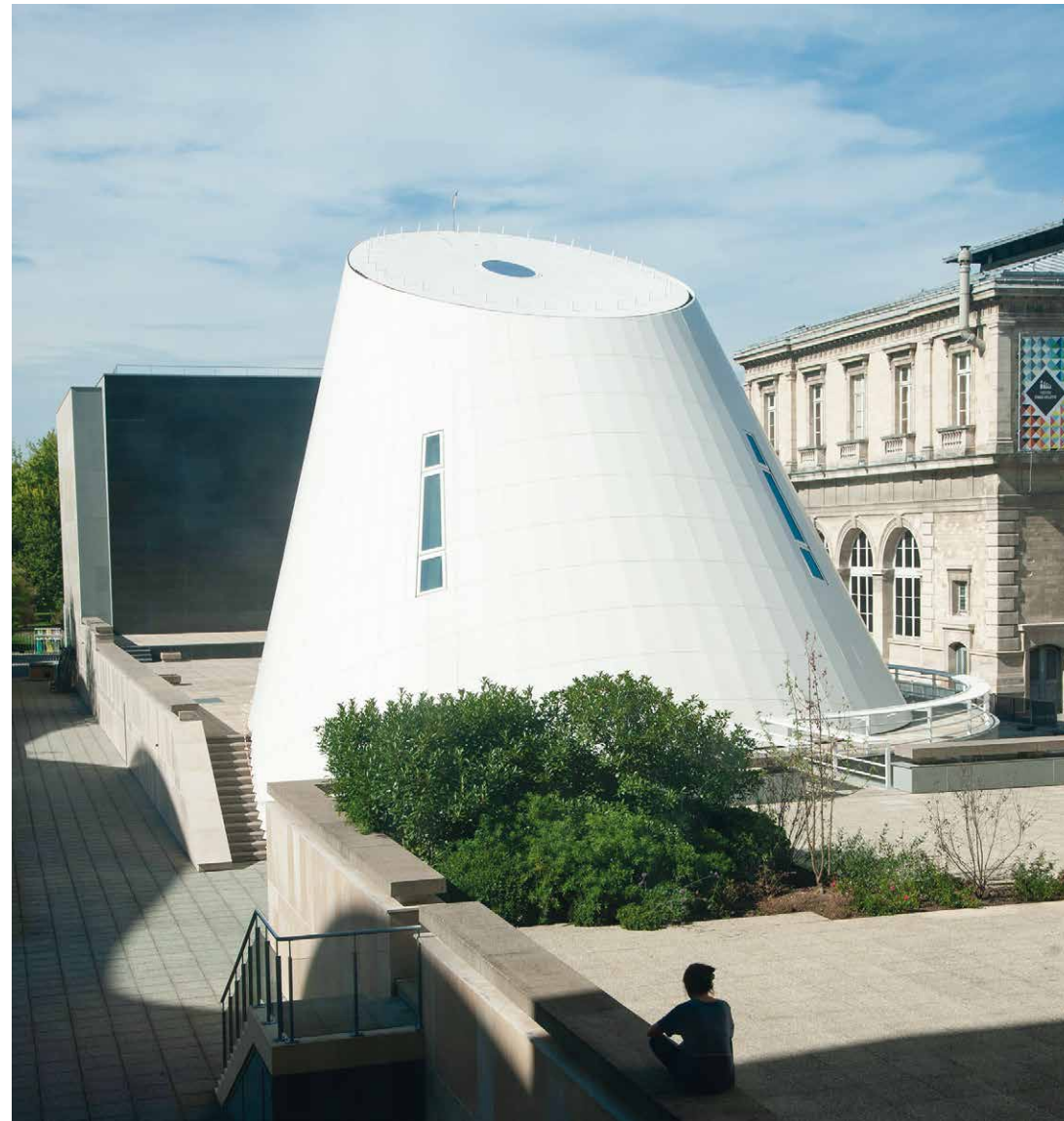
A total of 1,268 panels of Krion® Lux 6502 make up the unique façade of this hall in the shape of an inclined truncated cone at the National Higher Conservatory of Music and Dance in Paris. Photos: Ferrante Ferranti / CNSMDP.
