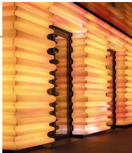
The changing lights on the façade are made possible by backlit plates of Krion ® 4102 Extreme Light Solid Surface.
