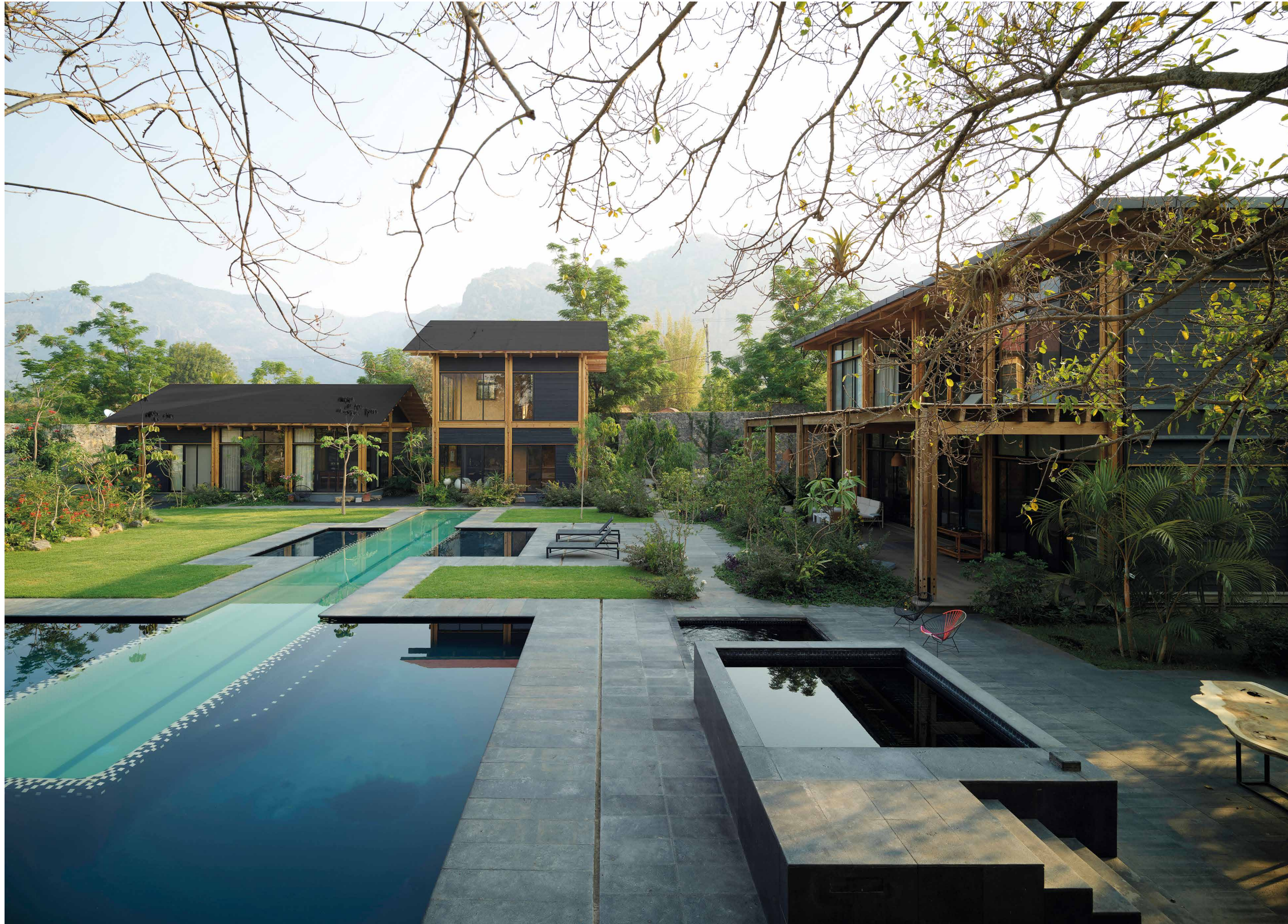
The prefabricated modules used for this project, located on a private property in Tepoztlán, have been built with pine from the Mexican state of Durango and have an original carbonised finish using the traditional Japanese technique of shou sugi ban .
