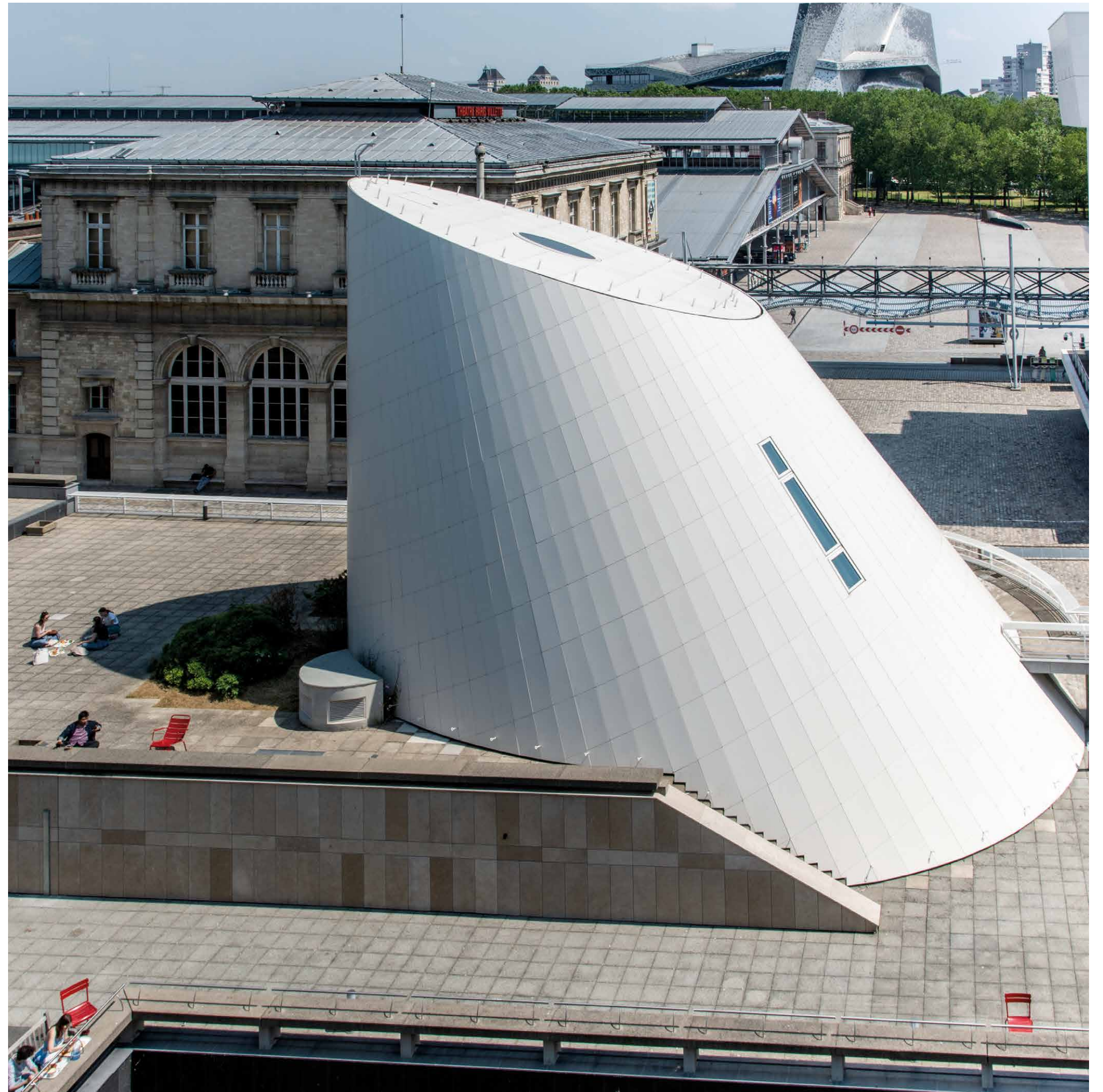
A total of 1,268 panels of Krion® Lux 6502 make up the unique façade of this hall in the shape of an inclined truncated cone at the National Higher Conservatory of Music and Dance in Paris. Photos: Ferrante Ferranti / CNSMDP.
